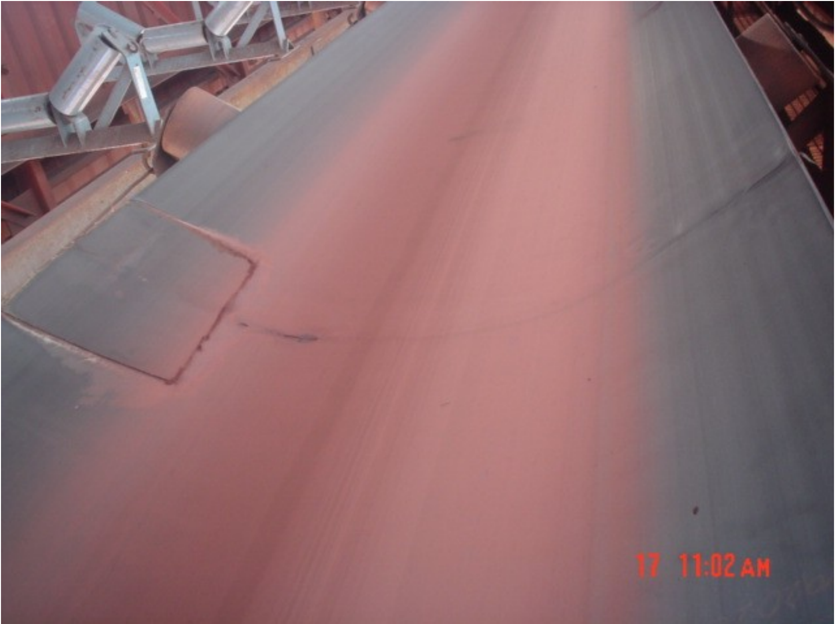
5F 1.55 conv. Top rubber & ply cut across the width
