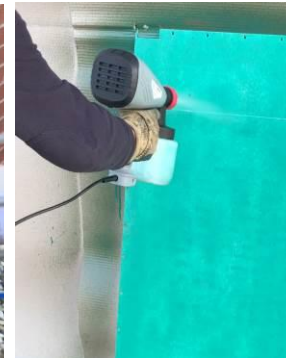
Apply with a pneumatic spray gun or an airless spray gun
