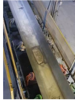
Crack repair with fabric reinforcement
