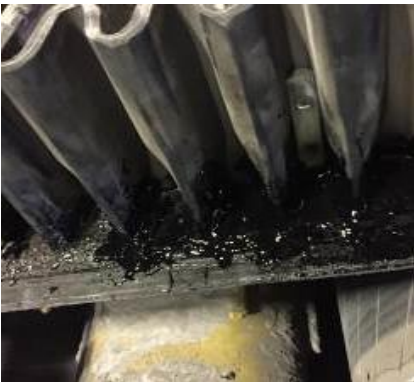
Sidewall belt repair
