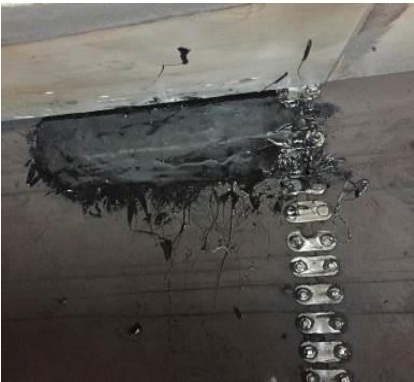
Rip repair beside bolt plate fasteners
