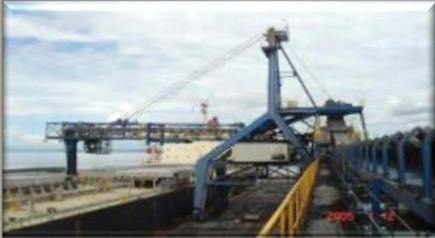
BALIK PAPAN COAL TERMINAL, (BCT) INDONESIA
