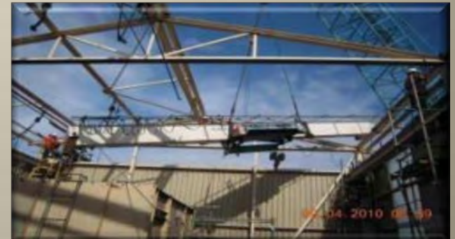
DISMANTLING OF EXISTING HOIST IN TRANSFER TOWER
