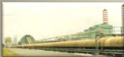
Power Plant Conveyor
