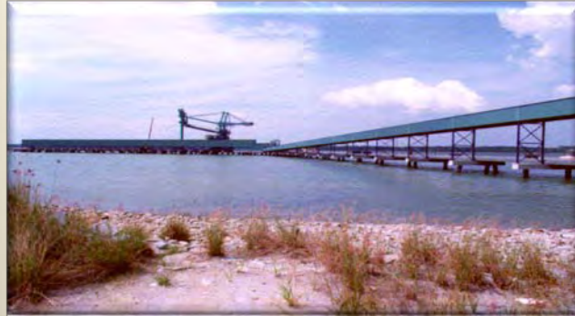
WEST PORT MALAYSIA
