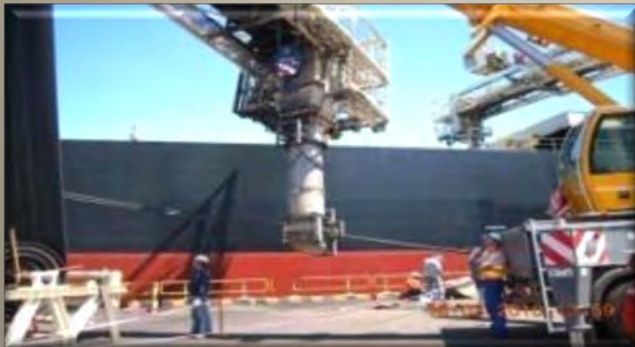
DISMANTLING OF EXISTING CHUTE OF SHIPLoader
