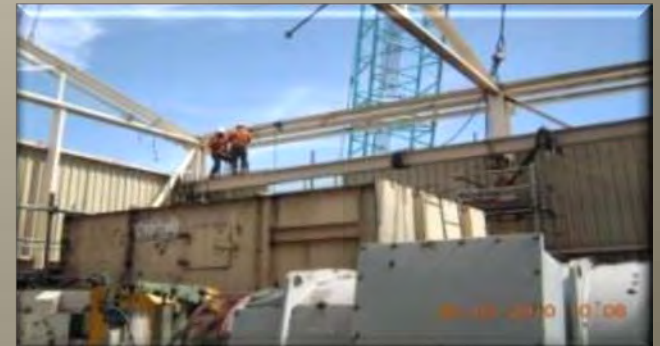
NEW HOIST ERECTION IN TRANSFER TOWER
