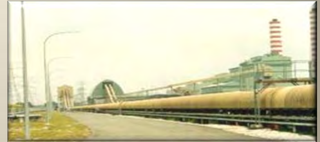
KAPAR POWER PLANT UPGRADE WORKS
