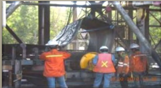
ERECTION OF NEW TAIL PULLEY FOR RECLAIMER CONVEYOR
