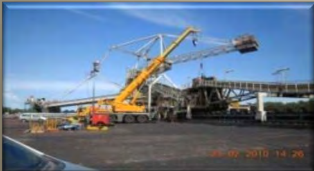
REPLACEMENT OF TRIPPER PULLEYS OF RECLAIMER
