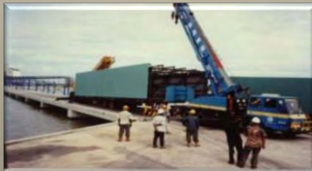
WEST PORT, MALAYSIA
