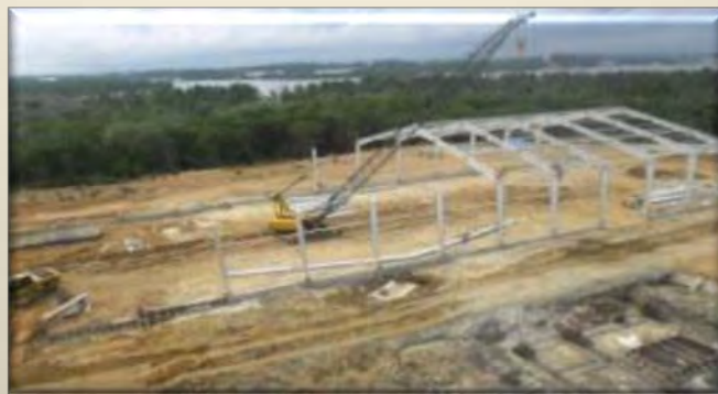
CLOSED COAL STOCK YARD CONSTRUCTION
