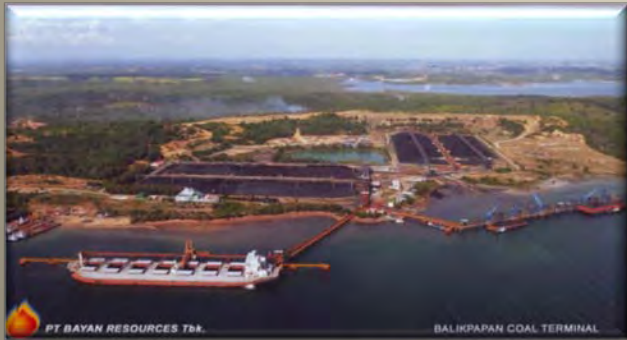
BALIKPAPAN COAL TERMINAL, INDONESIA
