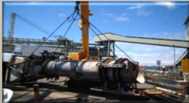
DISMANTLED EXISTING CHUTE OF SHIPLoader
