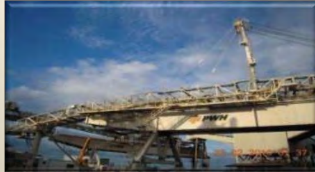
NORTH SHIPLoader BOOM & TIEROD REPLACEMENT
