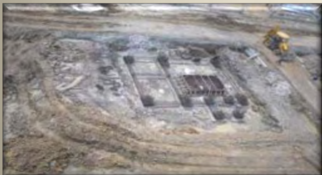
FOUNDATION FOR CRUSHER HOUSE
