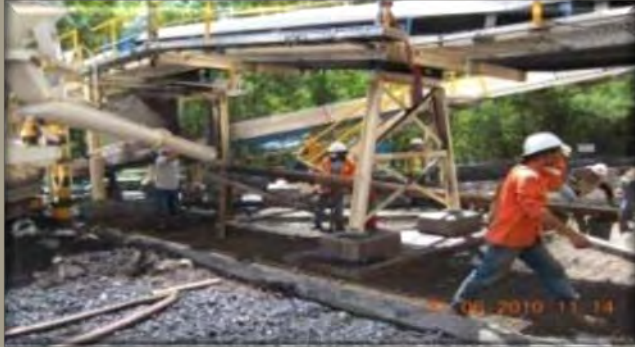
CIVIL WORK FOR SAMPLING PLANT
