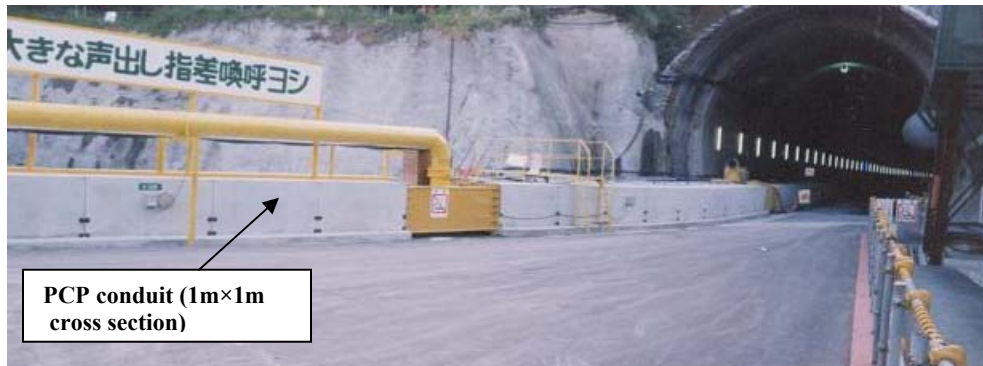
(a) Tunnel entrance
