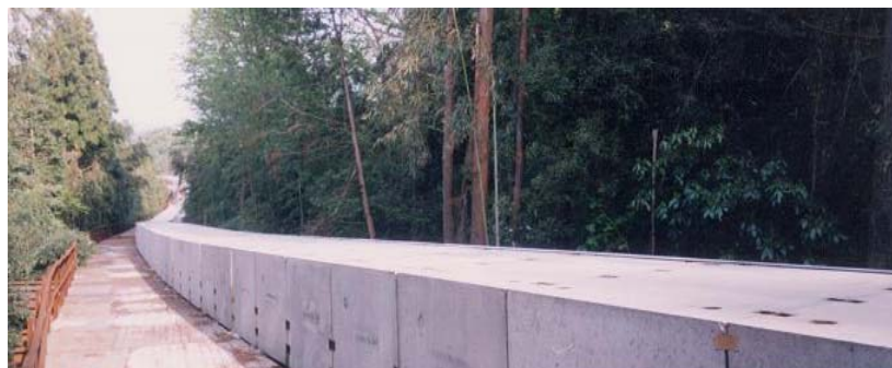
(b) PCP conduit extending outside the tunnel to the dumpsite
