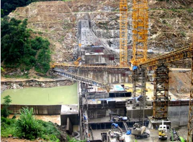
Dam project with 50m long conveyors using dual drives – 2 x 800M, 37kW
