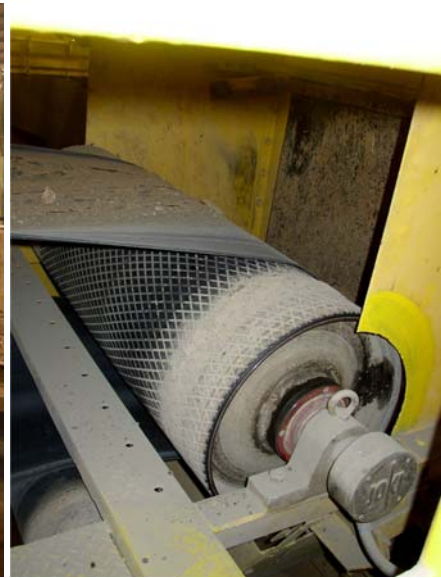
Cement – 500H installed in each bridge
