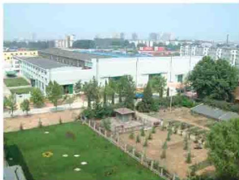
A corner of the manufacture workshop
