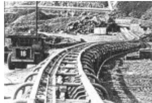
Fig.12. Alignment of the horizontal curve of the belt conveyors
