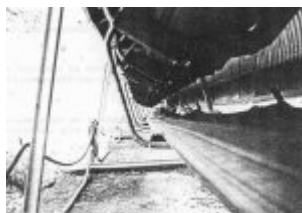
Fig.15. Idler frames of the return-side
