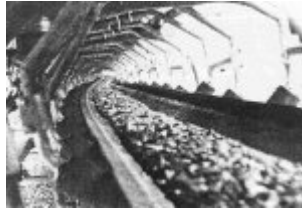
Fig.14. Belt travel of the loaded carry-side
