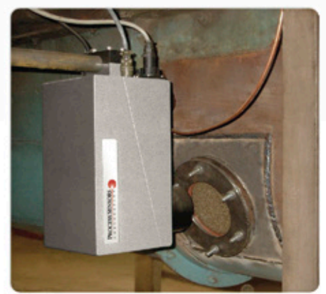
Moisture through sight glass
