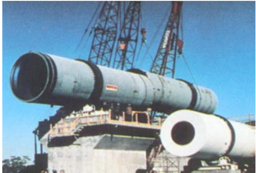
Field construction of Bartlett-Snow™ Rotary Dryer
