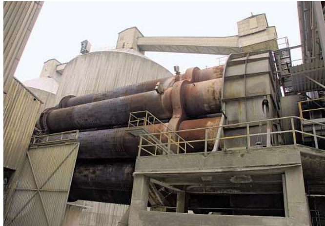
The rotary kiln which produces up to 3500 metric tonnes of cement clinker per day.
