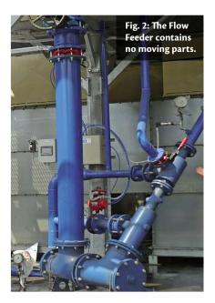
Feeder into the destination area. Once the dust level in the discharge hopper drops down to the minimum level, the equipment is shut down and waits until sufficient dust quantity is collected again.
