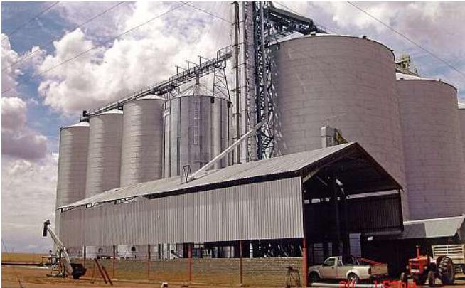
Fig. 2: The silo complex before the failure.
