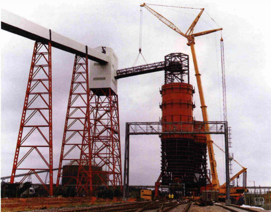
Fig. 4: Train loading facility during construction
