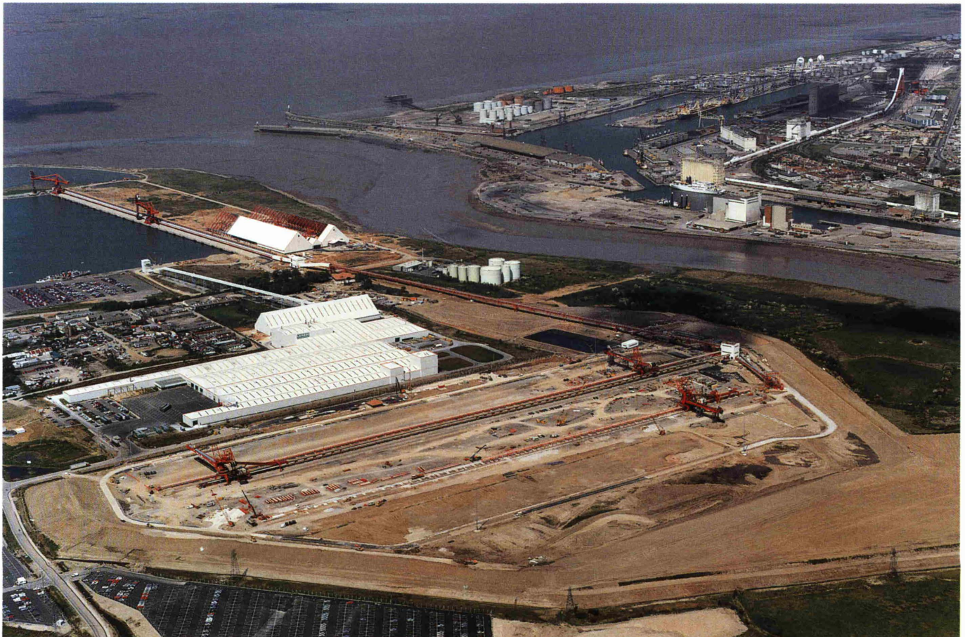
Fig. 2: Aerial view in the construction phase of Bristol Terminal with unloaders middle left, stockyard bottom centre and train loading facility top left
