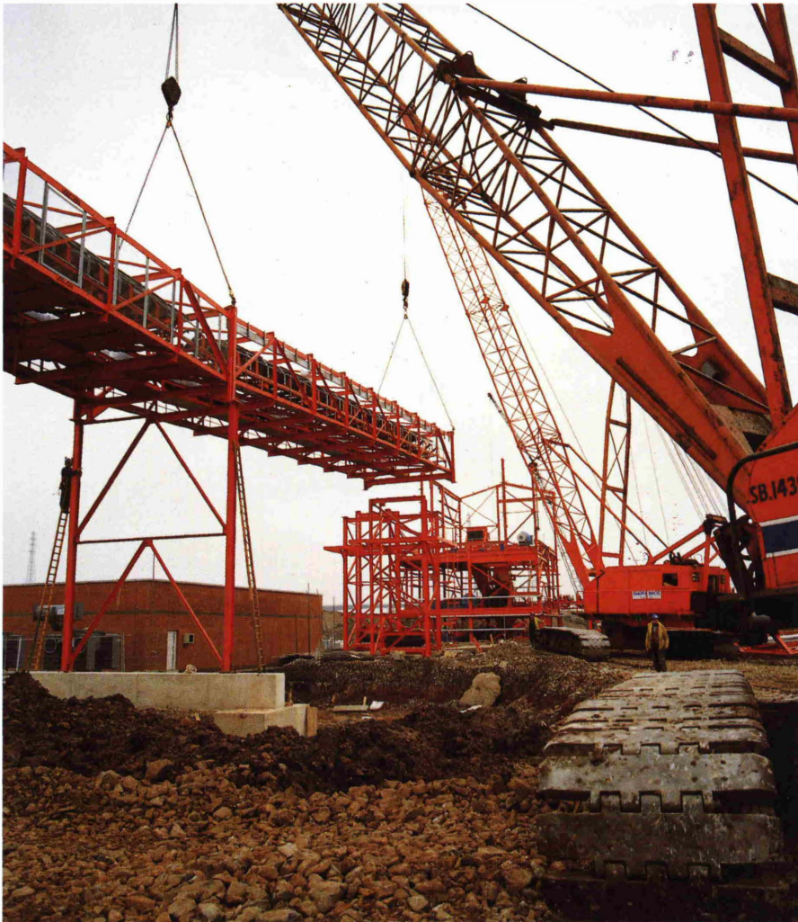
Fig. 3: Erection of double conveyor gantry with transformer bay in background
