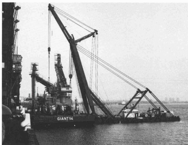
Fig. 2: Floating crane lifting the new coal unloader ashore at Kingsnorth
