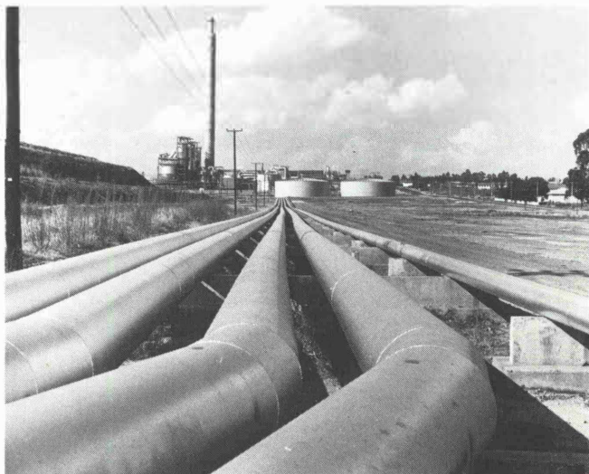
Fig. 1: Slurry pipelines and return water pipelines with acid plant and storage tanks in the background.
