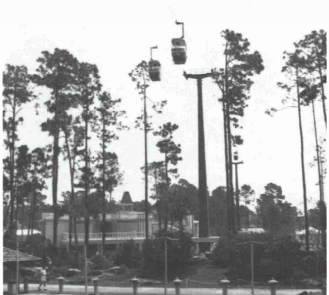
Fig. 1: Passenger-carrying ropeway, operating in an American amusement park, illustrates how the slender towers easily merge with the surrounding trees
