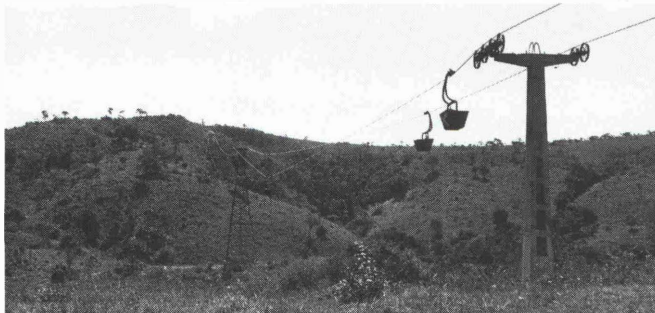
Fig. 3: Even on an open hillside ropeway towers are not easily visible to the casual observer
