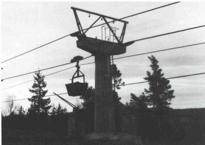
Fig. 2: Concrete towers are sometimes used to blend into the countryside
