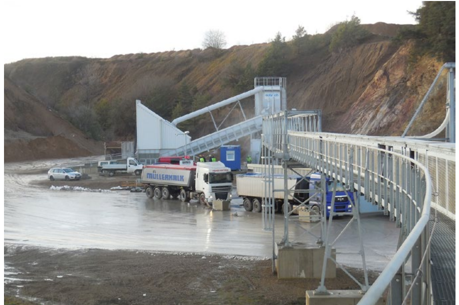
At the feeding station, clinker is transferred onto the pipe conveyor.
