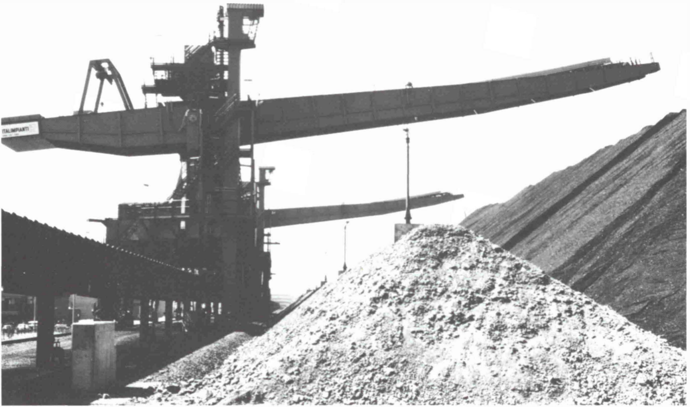
Fig. 6: 2 stackers served by 1 conveyor are part of the first multiple stacking system which eliminates waiting between trains. While 2 stackers stack coal unloaded by train and truck, the third is positioned to be ready for the next train arrival. Special berm protects runway from slumping coal.
