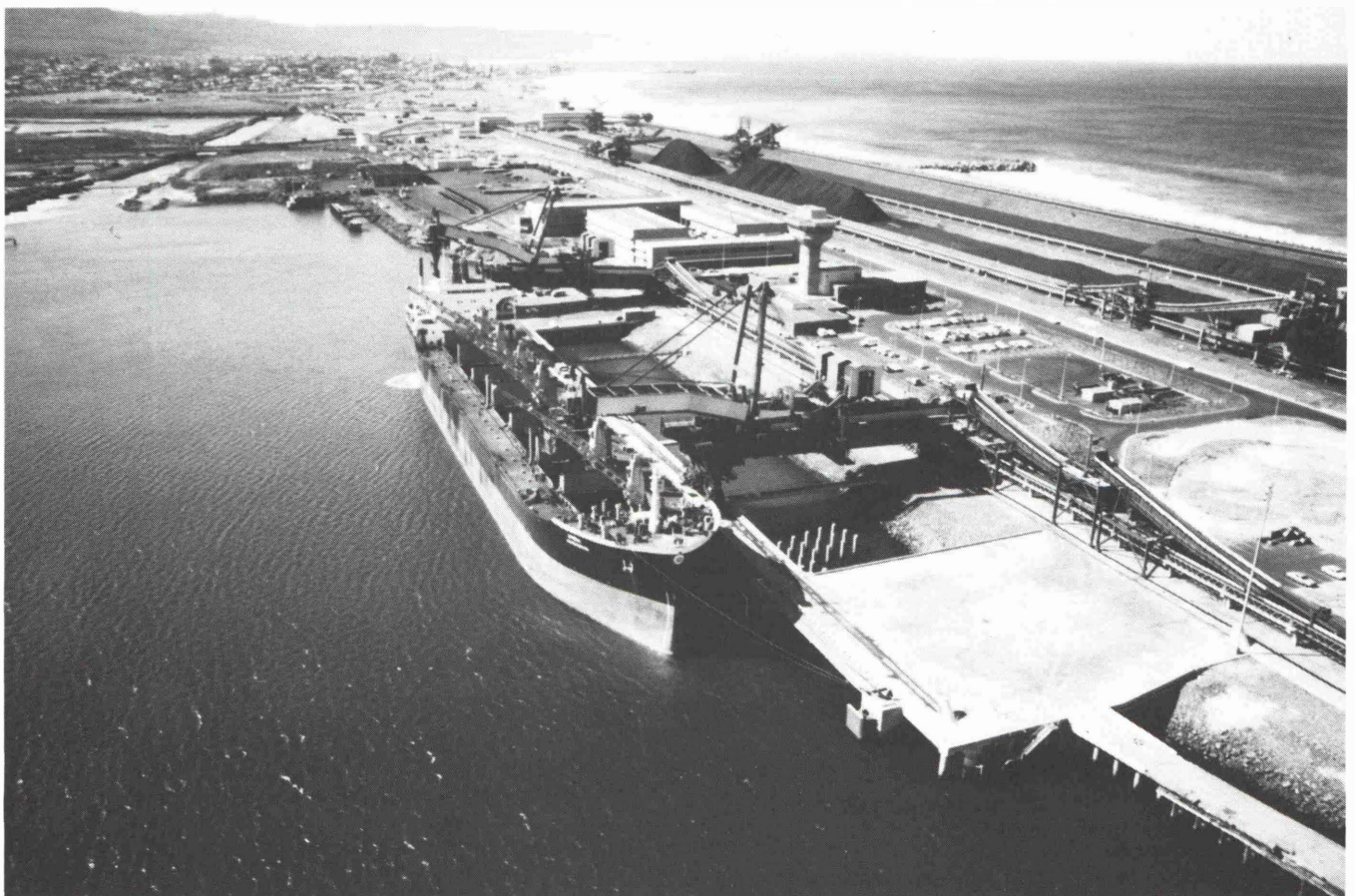
Fig. 15: Shiploaders are the first with launders that permit washdown and pumping away coal dust in slurry form. Solid decks at ends of the pier are washdown and maintenance areas. Public beach, golf course and residential areas are visible in background.
