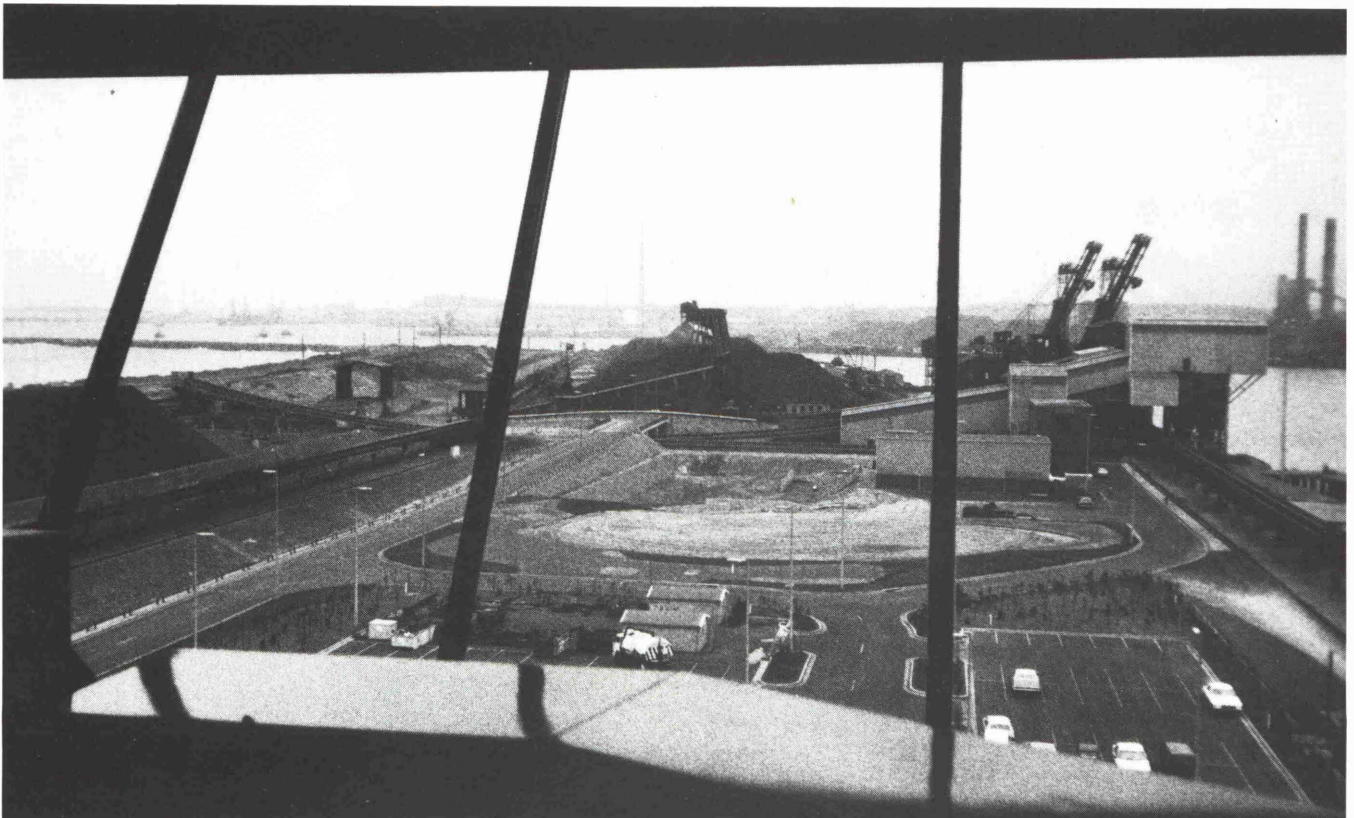
Fig. 9: View from shiploading control tower show switch bins used in conjunction with the dock conveyor and the recirculating conveyor for purging the system and automated reorganization of the stockpiles.
