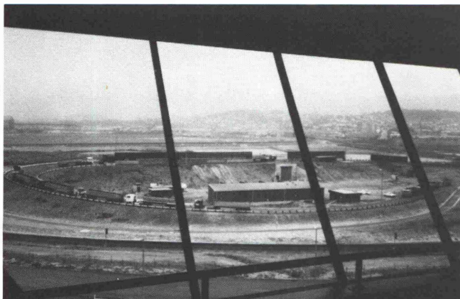
Fig. 3: View from receiving control tower of 3 lane highway on top of covered slot storage. Large door in the center is crane access to maintenance bay for 2,000 TPH rotary plows.
