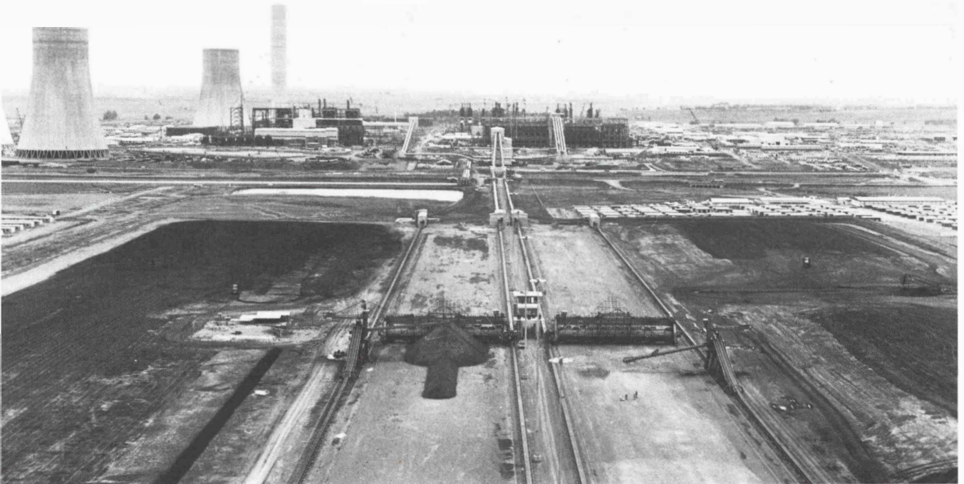
Fig. 8: The first coal stacked onto the 900 m long homogenizing beds at Sasol 2
