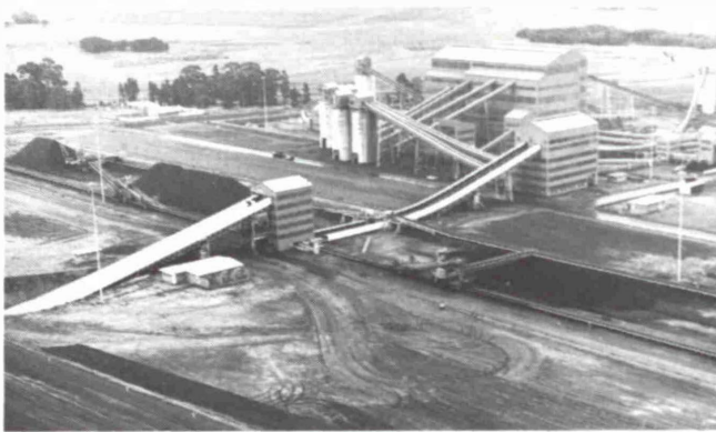
Fig. 12: Anglo-American's coal washing plant at Kleinkopje, with the homogenizing plants in the foreground. Note how easily the beds could be expanded in the future
