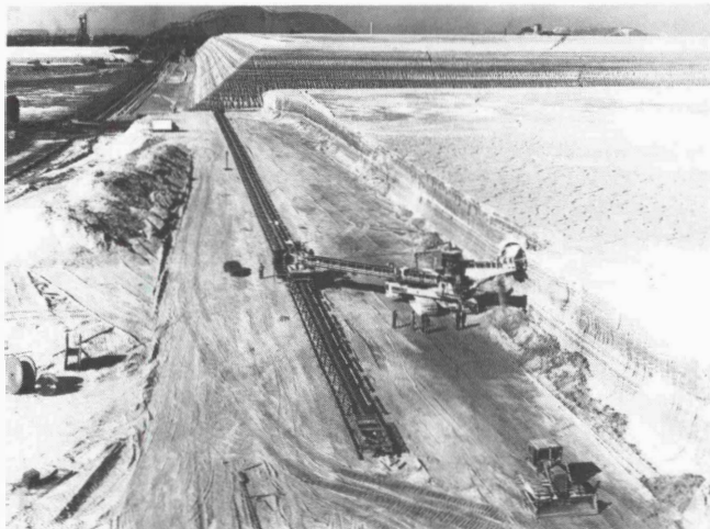
Fig. 4: View of the plant at the second cut
