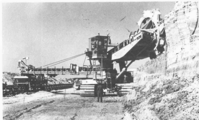
Fig. 5: Bucket wheel excavator while digging
