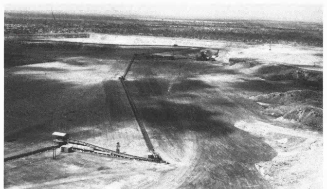
Fig. 8: In-pit crusher belt conveyor system
