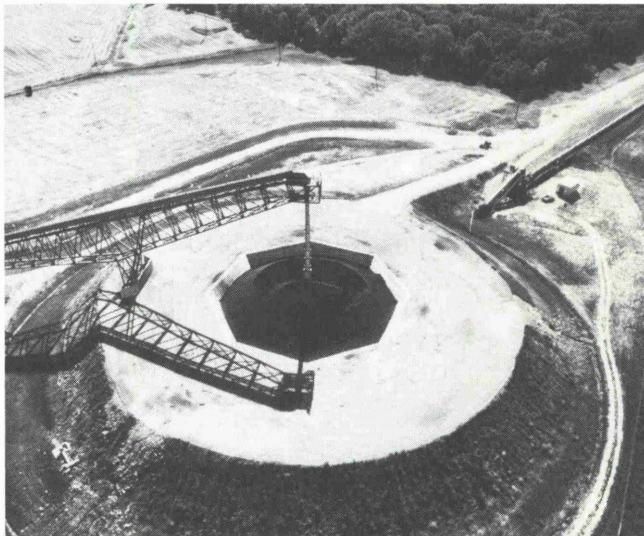
Fig. 5: "Glory-hole" type structures, built as octagonal inverted cones, are used as surge piles for nearby coal mines
