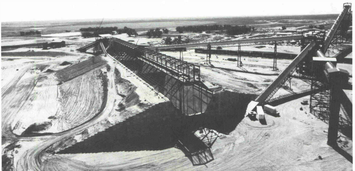
Fig. 7: Public Service Company of Colorado's Pawnee Generating Station has a 33,000-ton barn-covered slot with Reinforced Earth inclined (60°) sidewalls and vertical wingwalls. The structure, located at Brush, Colorado, has cast-in-place divider walls which accommodate coal blending during reclaim.
