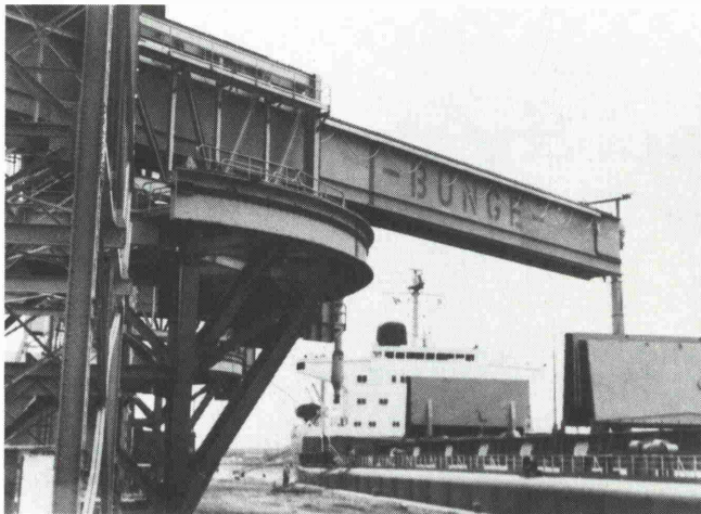
Fig. 2: View inside the shipping gallery
