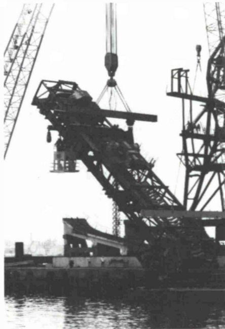
Fig. 9: Initial lifting of 300 ton boom assembly
