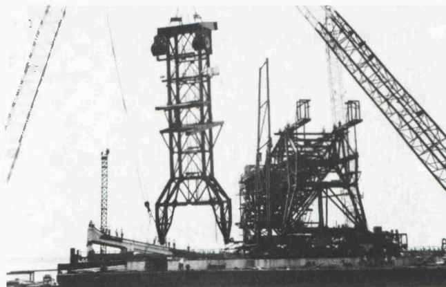
Fig. 5: Mast assembly suspended from Sun 800 barge mounted crane
