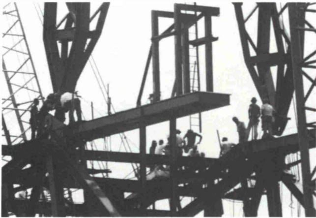
Fig. 8: Assembly of pin connected mast to bridge structure
