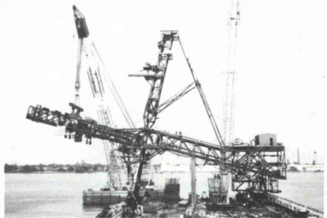
Fig. 12: Final connection of boom assembly to bridge and mast structure
