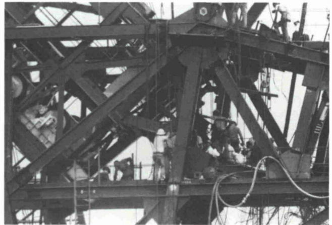
Fig. 11: Assembly of pin connected boom to bridge structure
