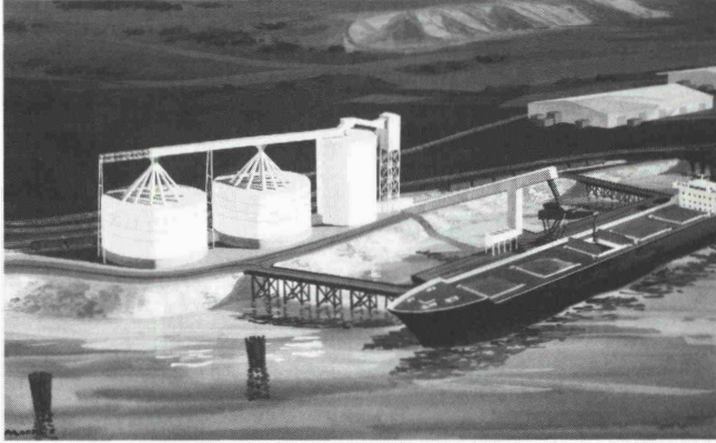
Fig. 4: Calcined Petroleum Coke Export Facility Longview, Washington
