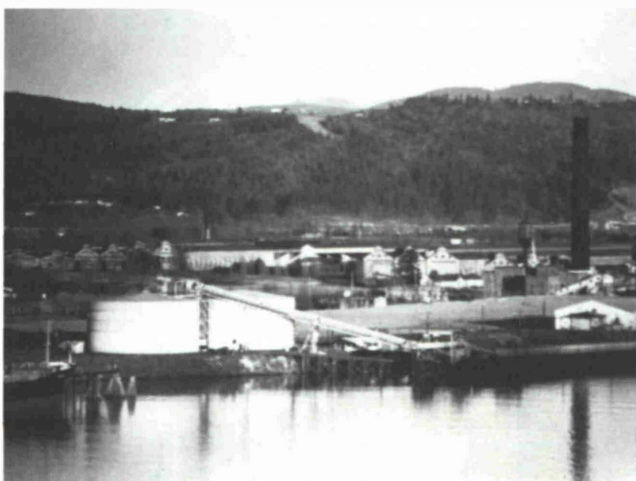
Fig. 1: Alumina Import Facility Longview, Washington
