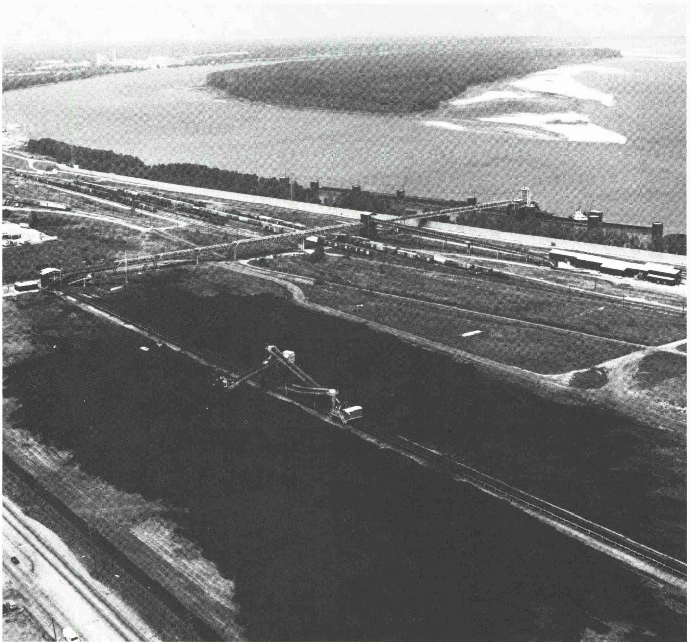
Fig. 3: American Commercial Barge Line Terminal, St. Louis, MI, can accept unit trains of Western Coal with a total ground storage of 500,000 tons handled by a stacker/reclaimer.
