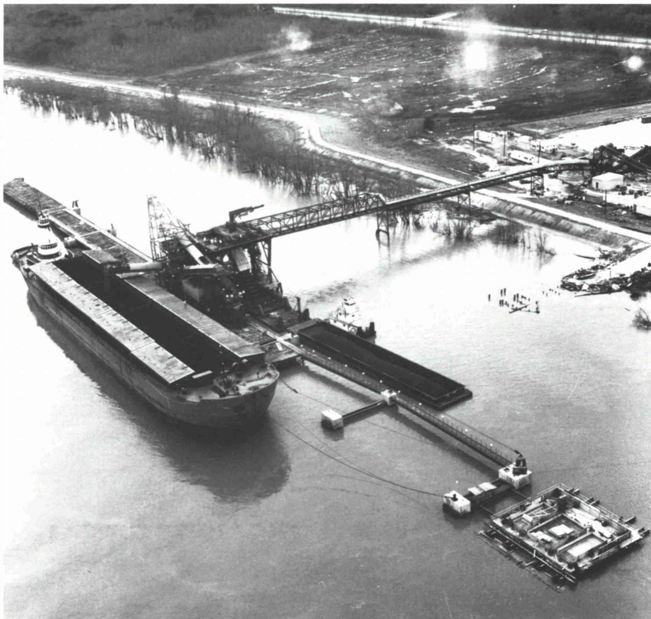
Fig. 4: International Marine Terminals Plaquemines Parish, LA facility. Although a phased construction program was planned, Dravo and IMT submitted all permit applications based on the maximum throughput level.
