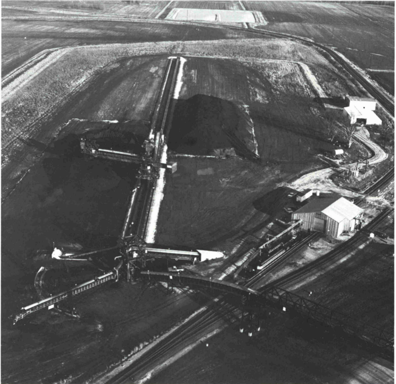
Fig. 14: An economical treating system can be phased to parallel the growth of the facility as shown at the IMT Plaquemines Terminal
