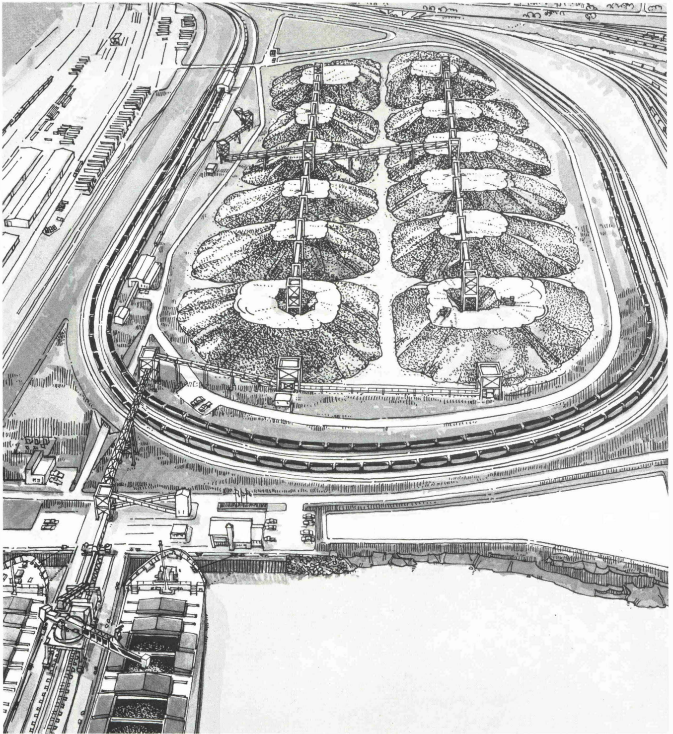
Fig. 1: Massey Coal Terminal, Newport News, VA. This coal transfer facility was designed by Dravo, who also managed construction. The facility has a tandem rotary car dumper / positioner system capable of unloading trains of random coal cars at the rate of 5000 tons per hour. The one-million-ton ground storage facility consists of overhead shuttle belt conveyors and gravity reclaim tunnels feeding directly to an 8,000 t/h traveling shiploader. This facility features an innovative computer-assisted control system designed to monitor each coal shipment from mine to ship including on-site unloading, storing, reclaiming, blending and shiploading. The annual throughput capacity of the site upon completion will be 10 to 15 million tons.
