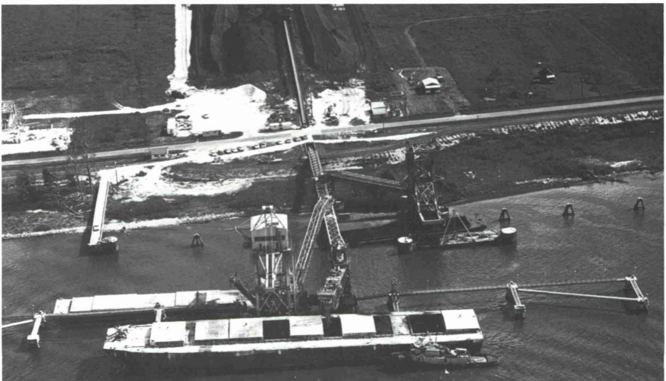
Fig. 13: This transfer terminal, operating since 1963, unloads coal with the Positioned-Twin Ladder Unloader at 3,000 t/h. Ground storage is accomplished with a 3,000 t/h Bucket Wheel Stacker/Reclaimer. Backhailed phosphate rock can be transferred with the 1,200 t/h Clamshell Bucket Unloader from the Gulf barge-to-river barge.
