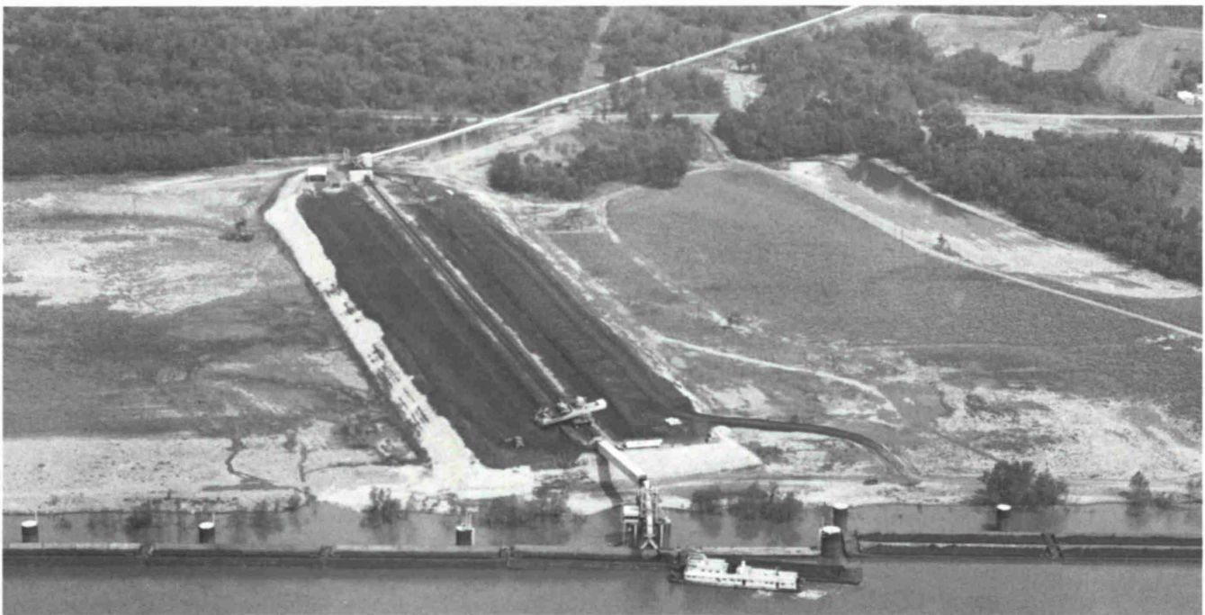
Fig. 7: River barge loading terminal. Coal is received by 1,200 t/h overland belt conveyor and directed to either ground storage or to waiting 15 barge tow for movement to destination.
