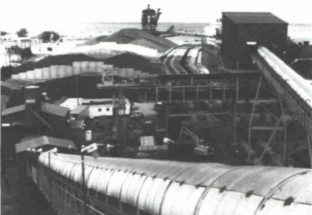
Fig. 3: Close-up of the Lorain Pellet Terminal installation showing hood covers over the conveyor belts to prevent dusting. The shiploader junction house is on the upper right and the pellet stockpiles are on the upper left.
