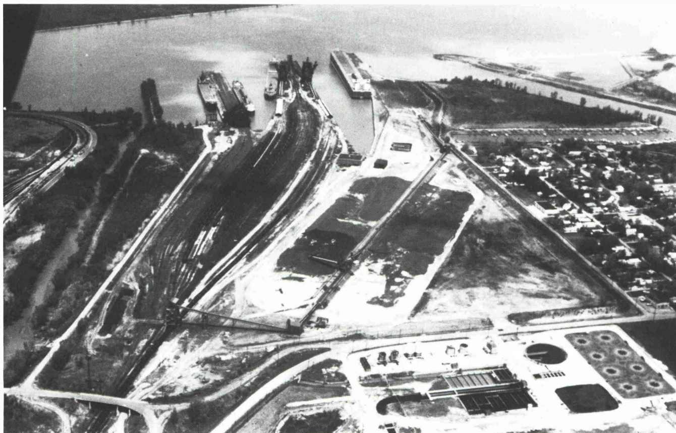
Fig. 9: Aerial view of the Toledo Terminal showing the 800,000 ton primary stockpile at the center and the dockside 100,000 ton surge pile near the top of the photo with a self-unloading ship discharging its cargo. The reclaim conveyor is at the center of the primary stockpile running towards the junction house to feed the transfer conveyor into the top of a surge bin for rail car loading.
