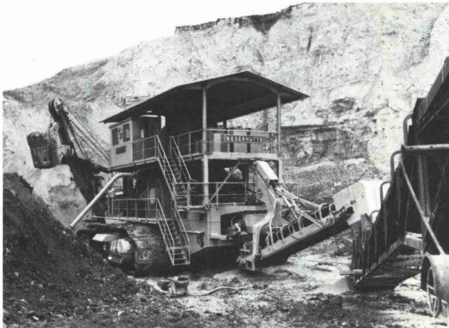
Fig. 3: Mobile crushing unit operating on difficult ground
