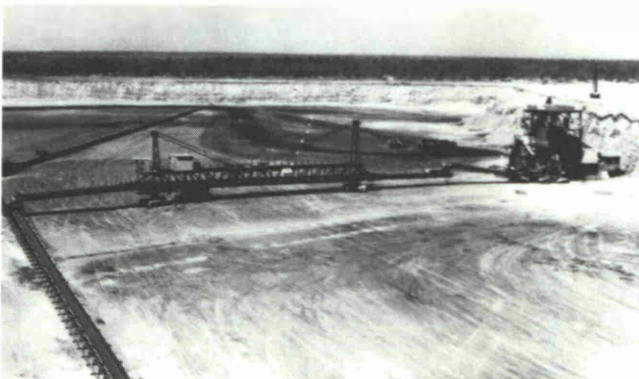
Fig. 1: In-pit crushing and conveying system
