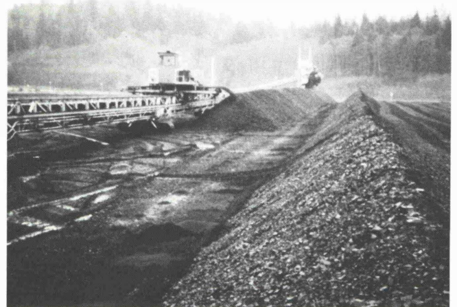
Fig. 10: 200 m RAHCO TMC in stack-out sequence
