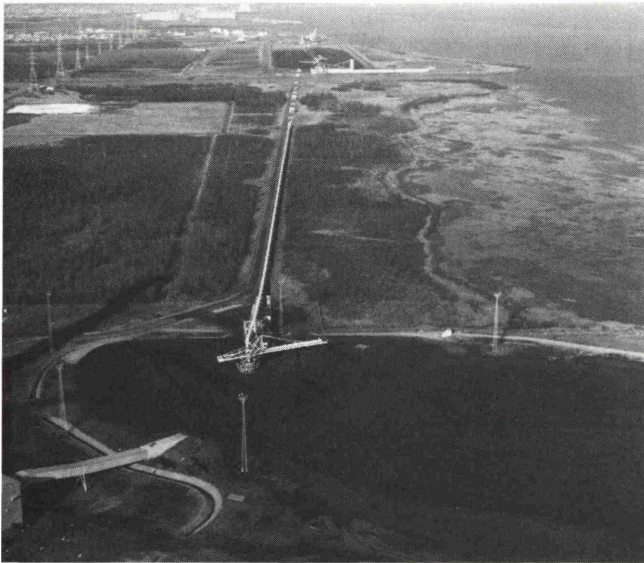
Fig. 1: View of the 2 km long overland belt conveyor extending from the trans-shipping terminal to the lignite stockpiles at the thermal power generating station
