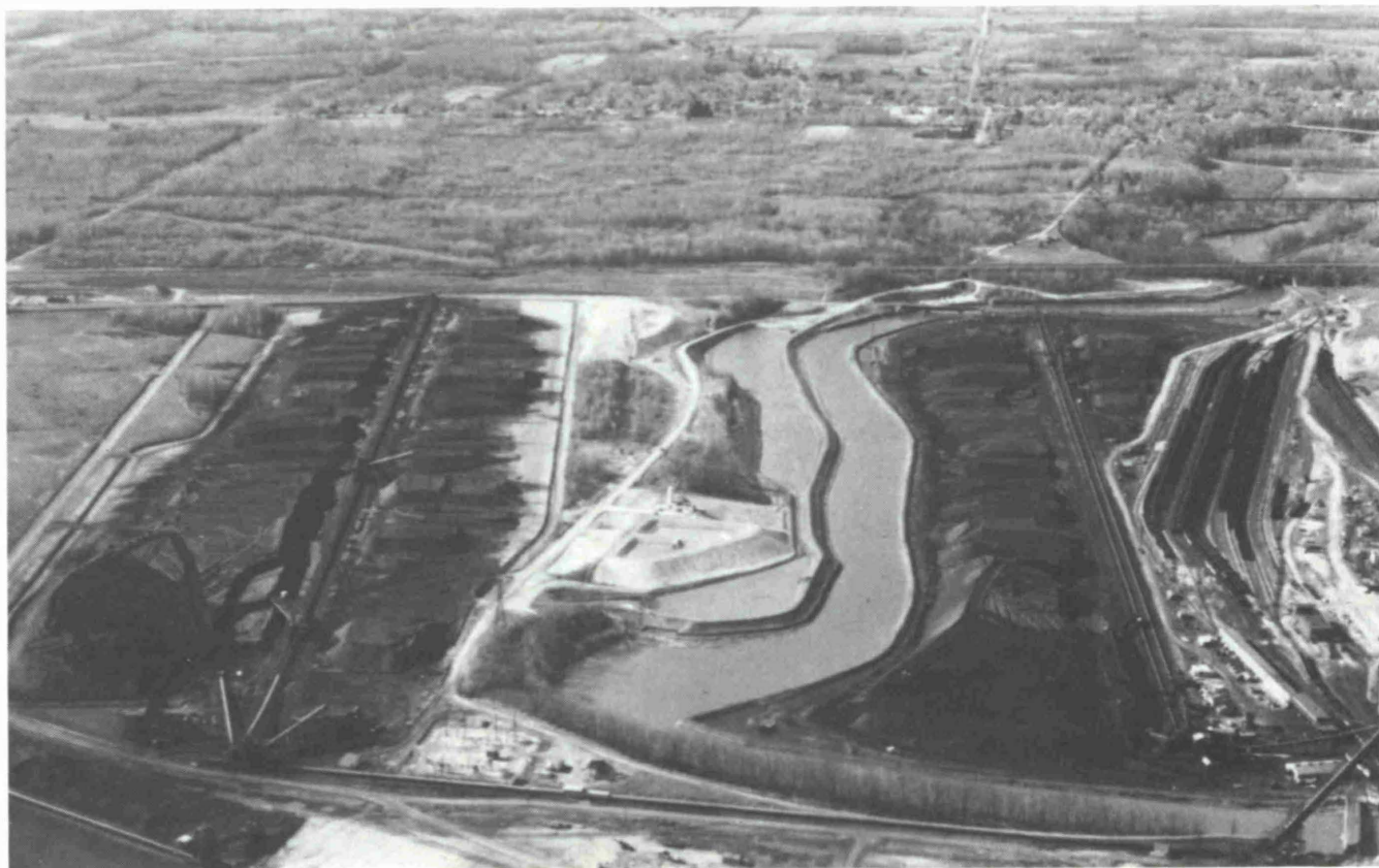
Fig. 7: New upper coal yard with 6,000 t/h single rotary dumper. Single yard belt has bucket wheel in front of stacker. One gravity pit is within reach of stacker, the other is fed by fixed stacker. The system is flexible, with above average reliability and low capital cost
