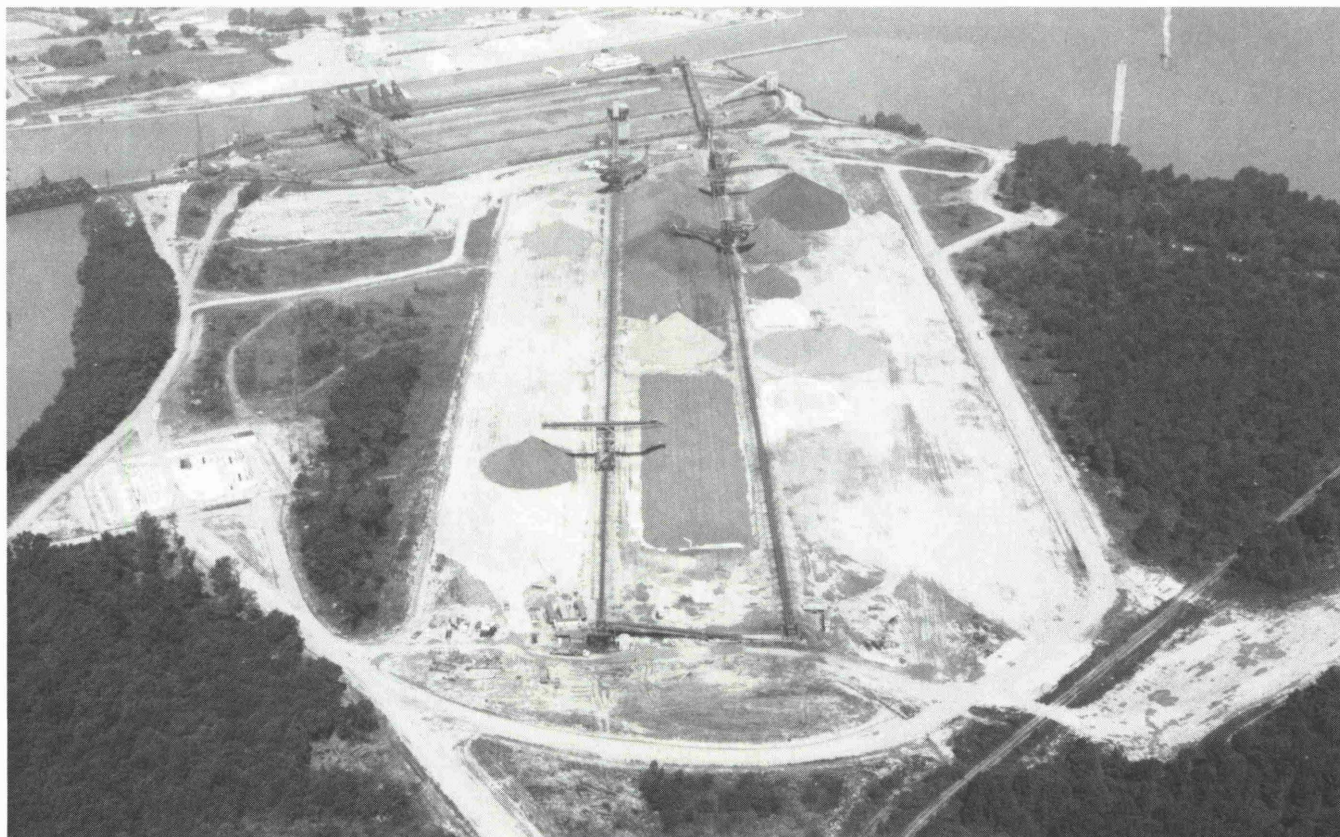
Fig. 4: Initial ore unloading terminal consists of 5 converted Hulett unloaders, 10,000 t/h stockpiling system, two bucket wheels and railroad loadout for random cars
