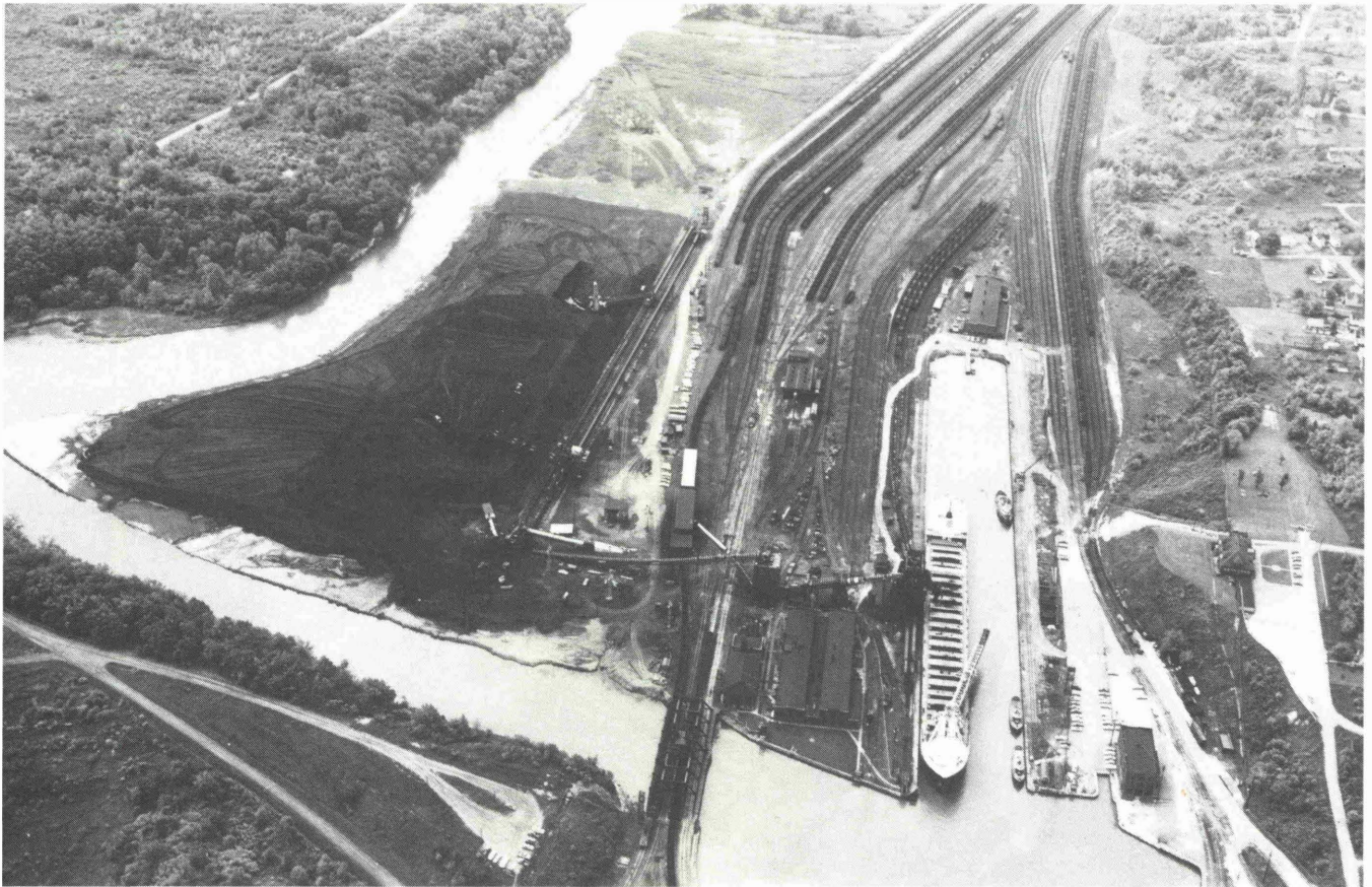
Fig. 1: Coal terminal, initial phase. Existing high rise dumper is converted to 7,000 t/h shiploader. Surge bin in front of loader can be fed at 6,000 t/h, with 3,000 t/h available from railroad, gravity pit or bucket wheel
