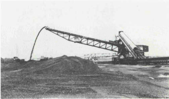
Fig. 9: Yard conveyor stacker with bypass
