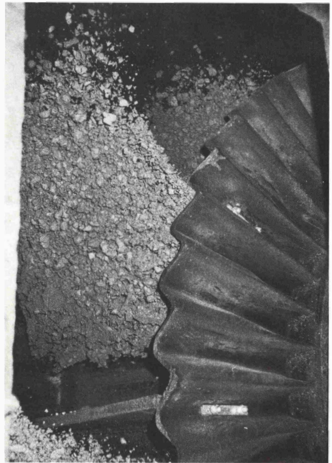
Fig. 14: View onto the discharge parabola during first unloading on May 28, 1982 with crushed limestone. Very clearly the photo shows the smooth removal of the wet limestone from each pocket. Due to the discharge by means of centrifugal force, it is ensured that no material is returned. Current requirement for the system while running without material: approx. 575 V 50 Amps (Amp.) and under full load approx. 160 Amps.
