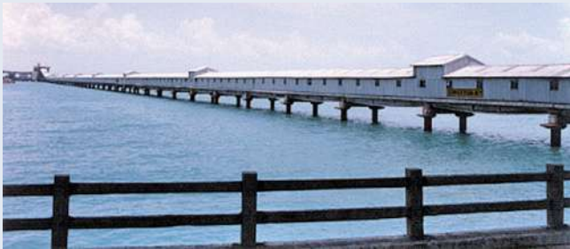
The conveyors which transport the coal to the power plant are routed through the sea for most part of the distance.
