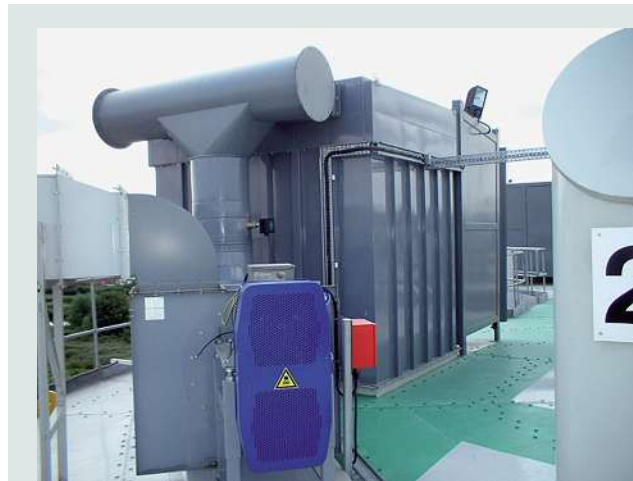
Fig. 2: Filter installation at the silo top, Combifab fan in foreground.
