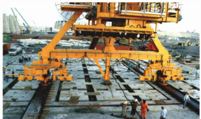
Fig. 1: Loading of a continuous ship unloader by using the 'Air Cushion' skidding system
