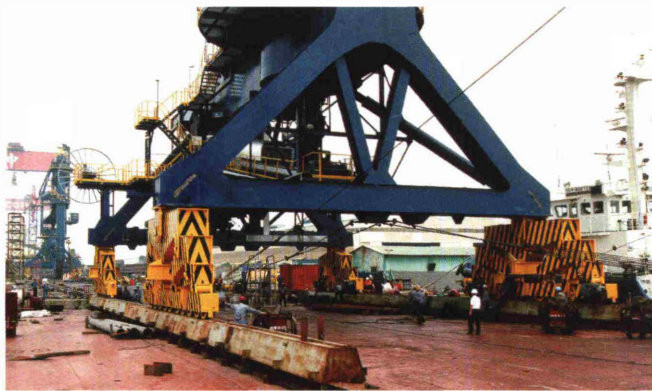
Fig. 4: Loading of a continuous ship unloader on own wheels
