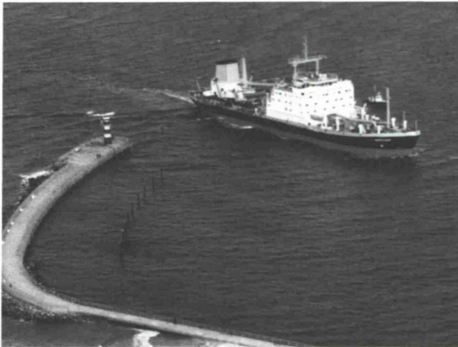
Fig. 4: Hopper suction dredger
