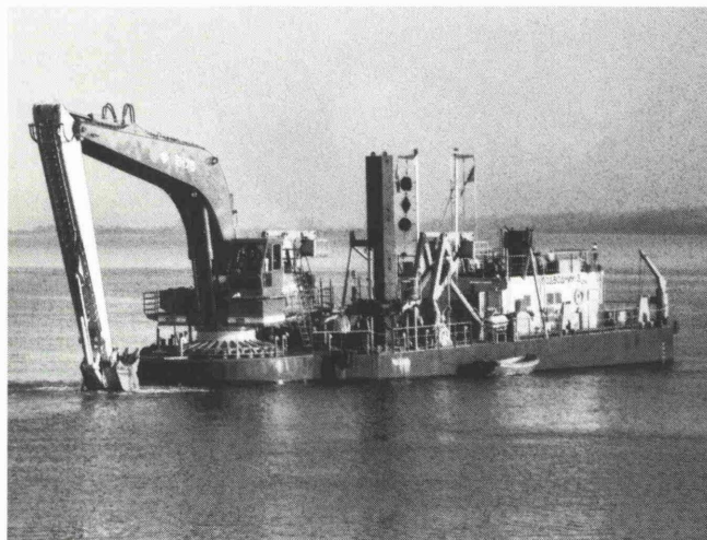
Fig. 2: Pontoon-mounted hydraulic backhoe as bucket dredger
