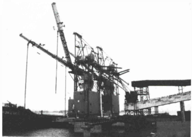
Fig. 4: Unloading from barge to dockside installation
