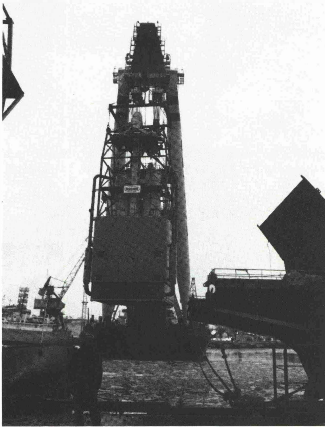
Fig. 1: Re-erection of central part of unloader onto pontoon
