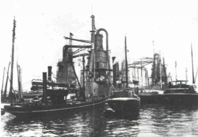
Fig. 1: Older steam discharging plant in operation
