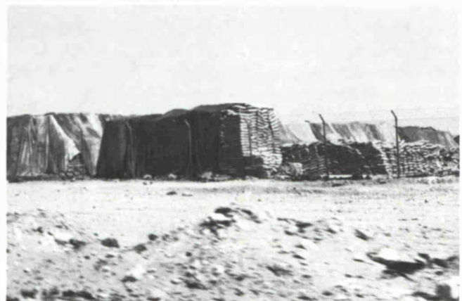
Fig. 8: Bagged cement stored in the harbour of Dammam (open air store; 1978/79)
