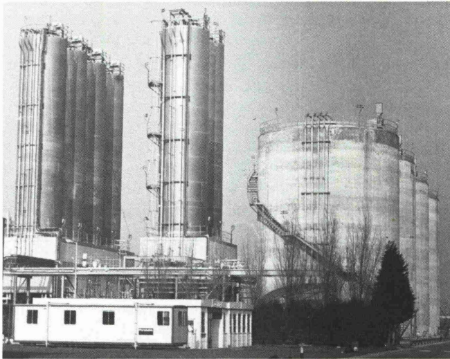
Fig. 3: View of silo installation
