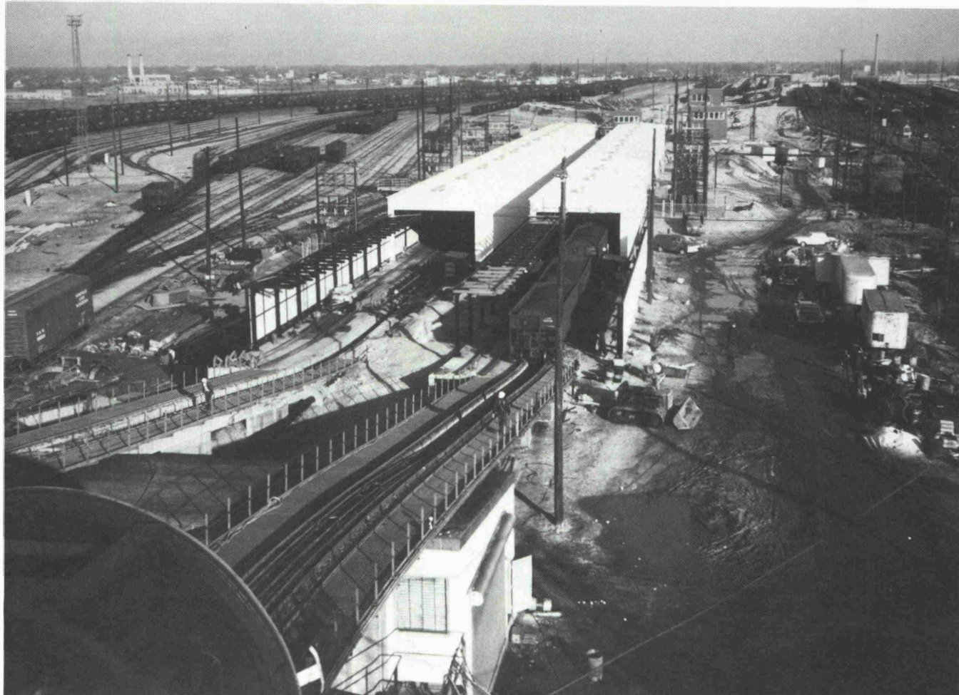
Fig. 4: A gravity feed system (background) to a barney (foreground)
