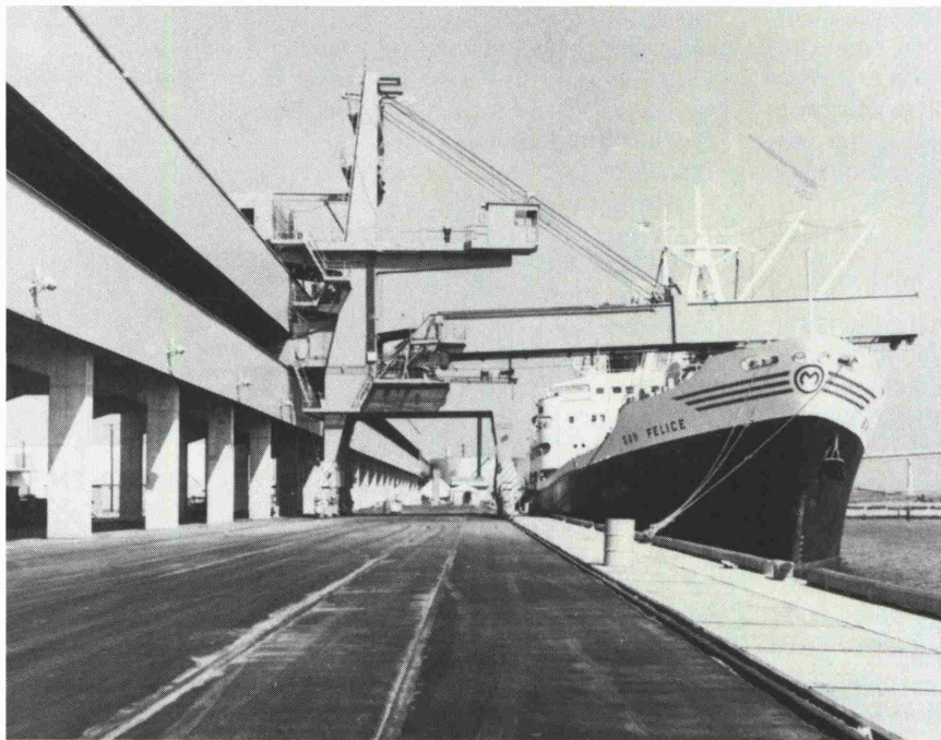
Fig. 2: Traveling tripper and dock conveyor of Soros design, with enclosed C gallery for improved environmental protection, now handling coal at Morehead City, NC, USA
