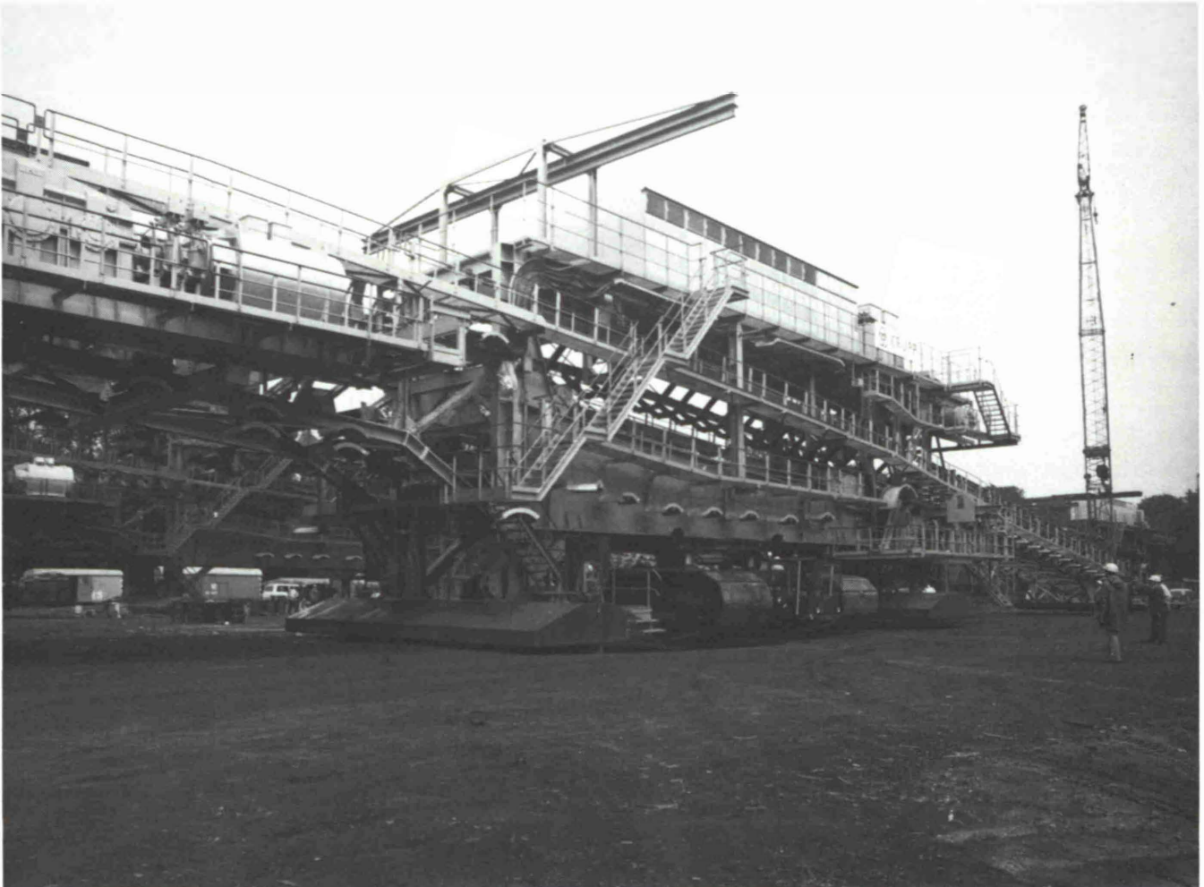
Fig. 2: A 4 x 2,000 kW conveyor drive unit being moved by a crawler-mounte
