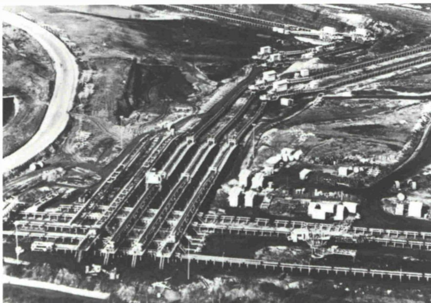
Fig. 11: Conveyor distribution point with extending conveyor heads
