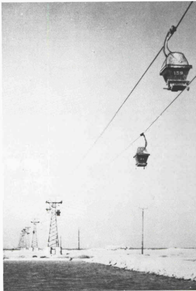
Fig. 3: Monocaber ropeway in Bahrain for transporting alumina from a jetty some 5,000 m offshore to an aluminium smelter inland.
