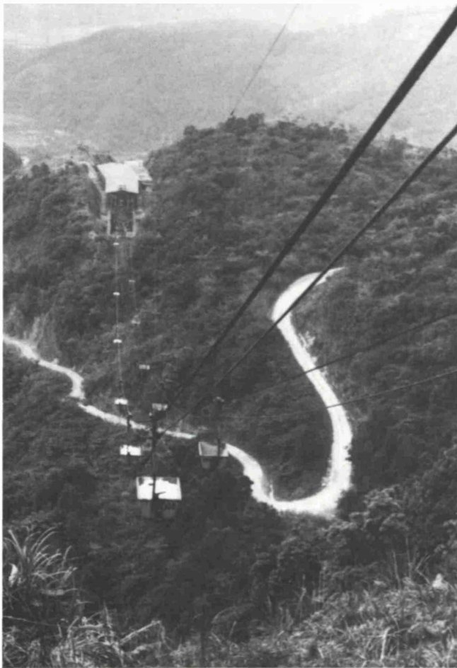
Fig. 4: Ropeway in Taiwan for transporting 420t/h of limestone from quarry to the cement factory.
