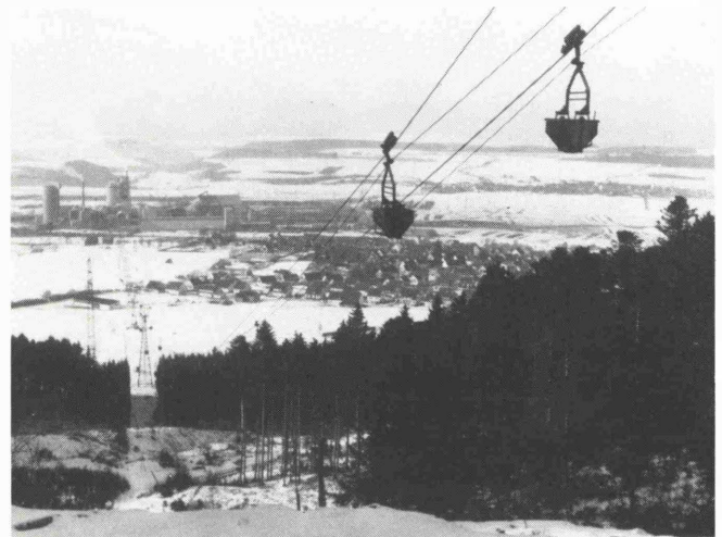
Fig. 1: Economic operation is an important feature of the bicable ropeway serving Portlandzementwerk, Dotternhausen, in the Federal Republic of Germany. Travelling downhill at 4.25 m/sec, the buckets — each loaded with 1665 kg of limestone — develop surplus power which is controlled by a 250 kW drive/brake gear, the electric motor of which acts as a brake.
