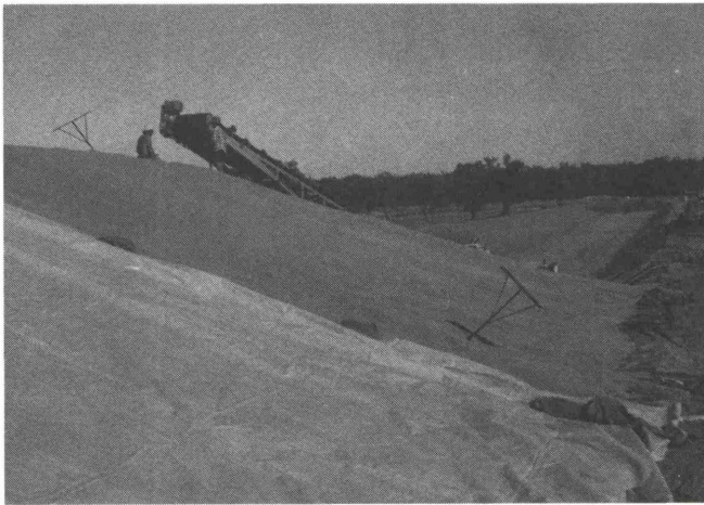
Fig. 1: Bunker showing the grain stockpile partly covered by "CANVACON"
