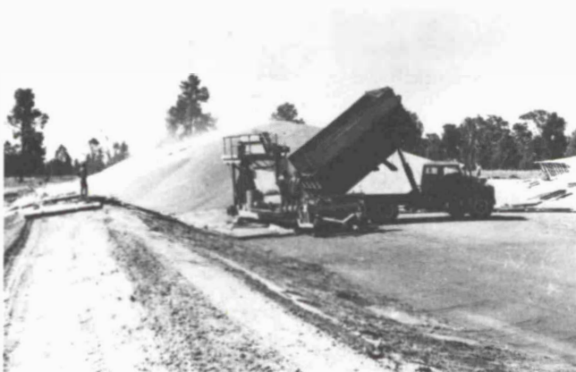
Fig. 2: PVC above-ground storage
