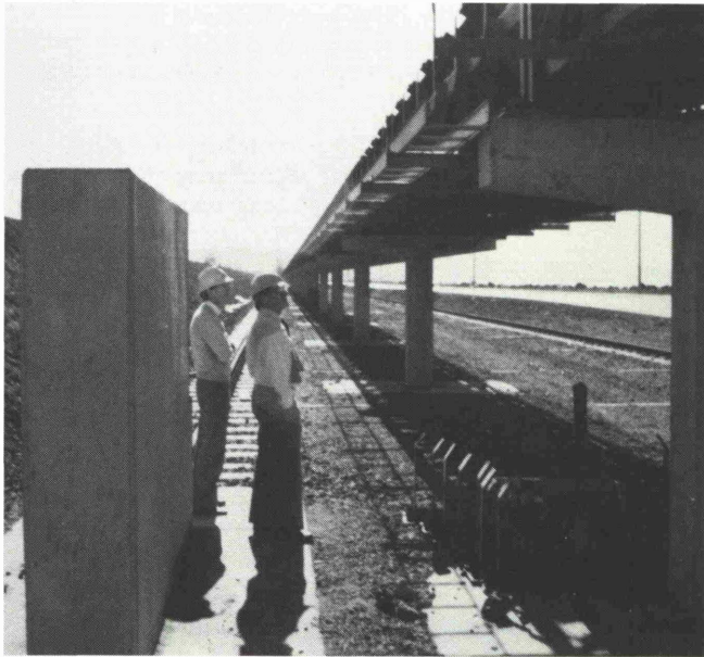
Fig. 6: Yard conveyors are on concrete posts to facilitate clean-up. Side berm protects against "slumping"
